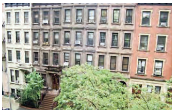
Is it awkwardly cropped? There could be a construction site next door.
